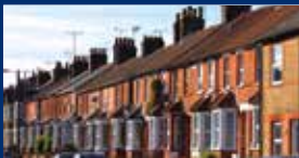
Micro-grid applications across housing estates, commercial developments and campuses
