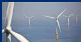
Conversion of hydrogen energy storage from renewables
