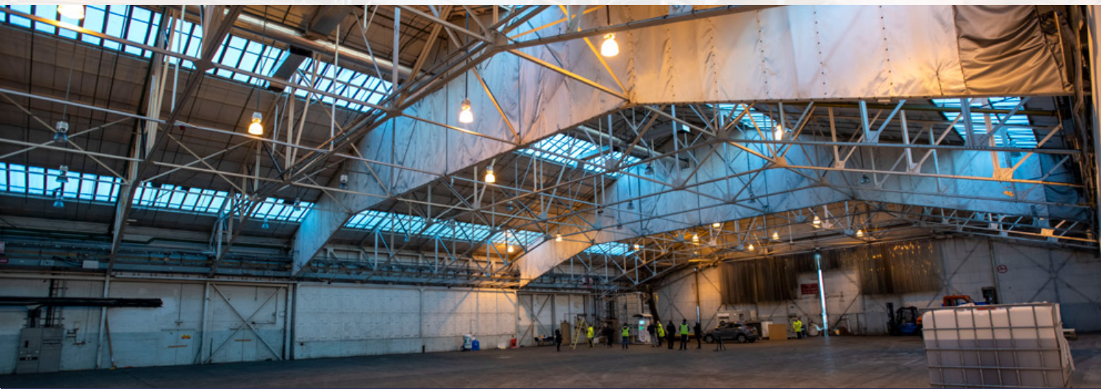
New Assembly & Commissioning Facility at Dunsfold prior to fit-out works, January 2021
