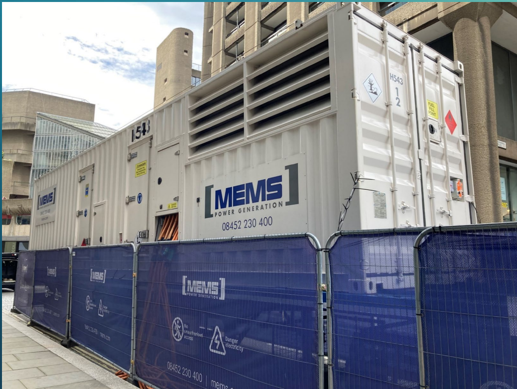
1MW Diesel Generator Operating Outside the Barbican in April 2024
